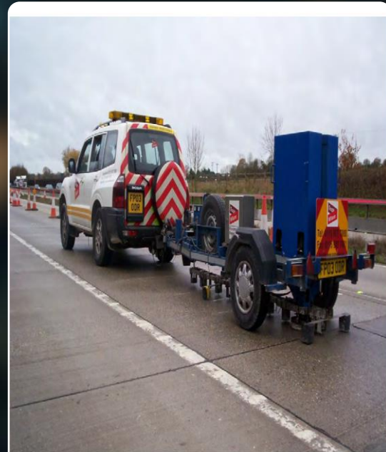
Figure 2.10 FWD undertaking concrete joint testing
